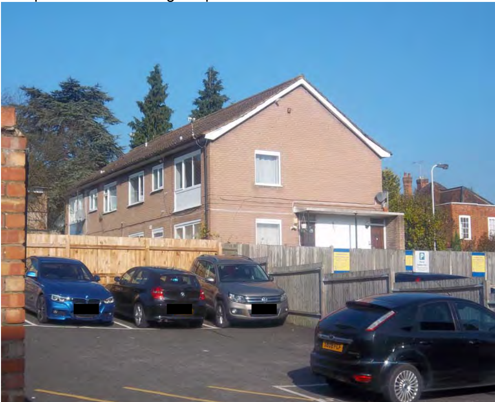
Existing windows at ground and first floor of Ray Gardens
